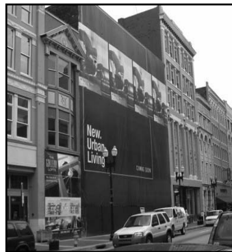
The J.C. Penney Building
